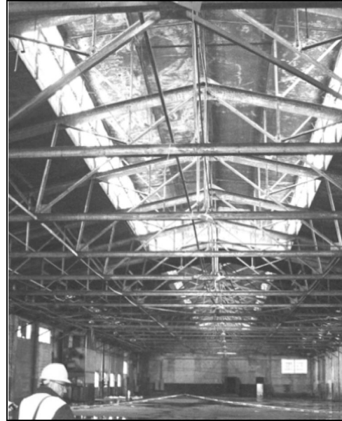
Long span trusses and light monitor
