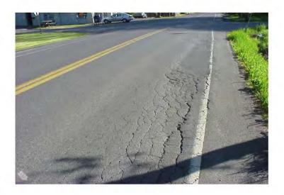
The longitudinal crack in this photo qualifies as alligator cracking even though it lacks the interconnected cracking. The crack is in the early stages of development, but still represents a load-related distress because it occurs in the wheelpath.
