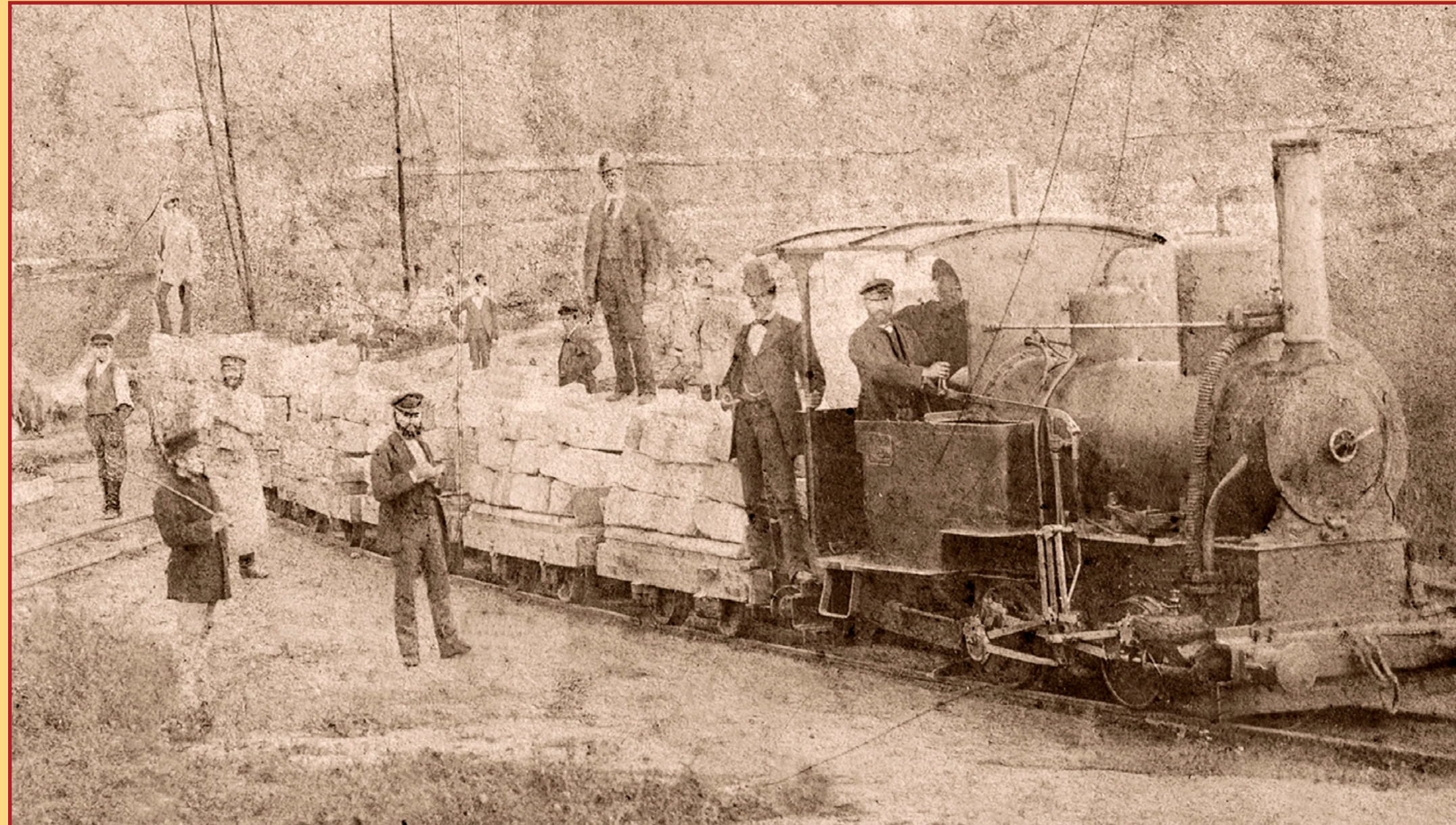
Fragment of a circa-1860's photo showing the Quarry Railroad car loaded with cut marble at the Quarry Wharf on the Hudson River. COURTESY OF THE HASTINGS HISTORICAL SOCIETY
