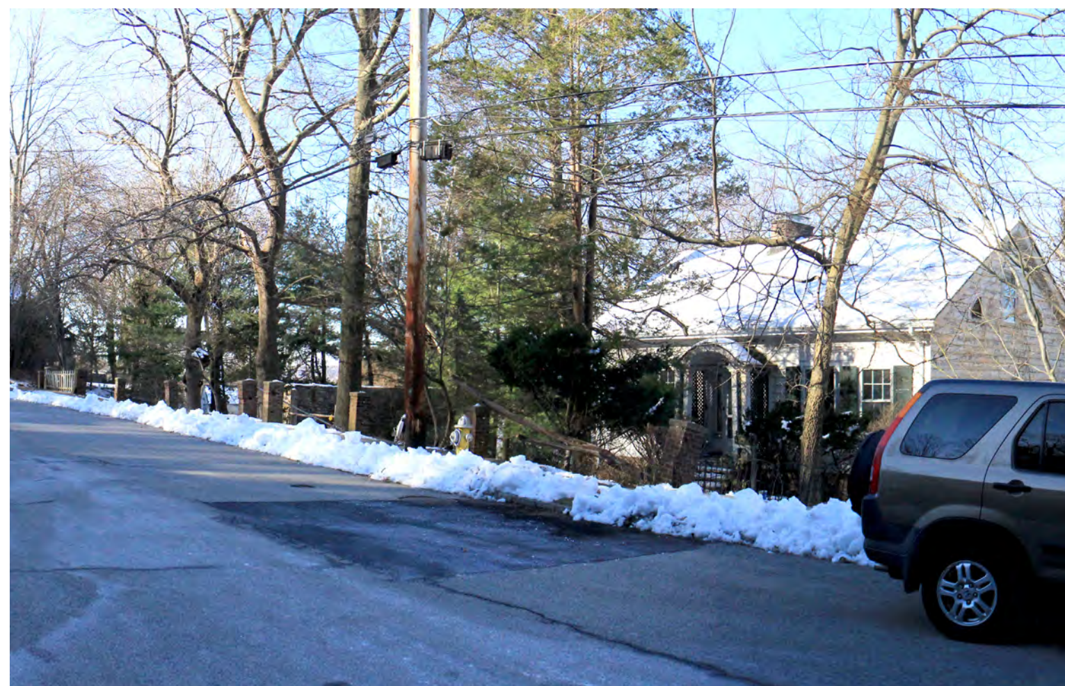
EXISTING: VIEW B (FROM STREET FACING SOUTH)
