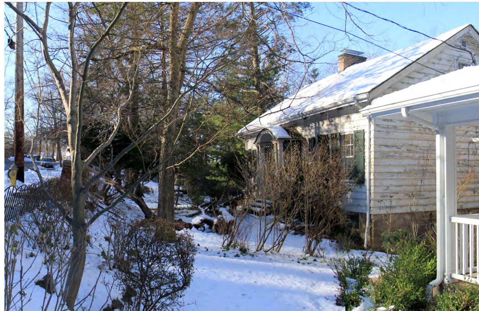
EXISTING: VIEW A (FROM 83 PINECREST PARKWAY FRONT YARD)
