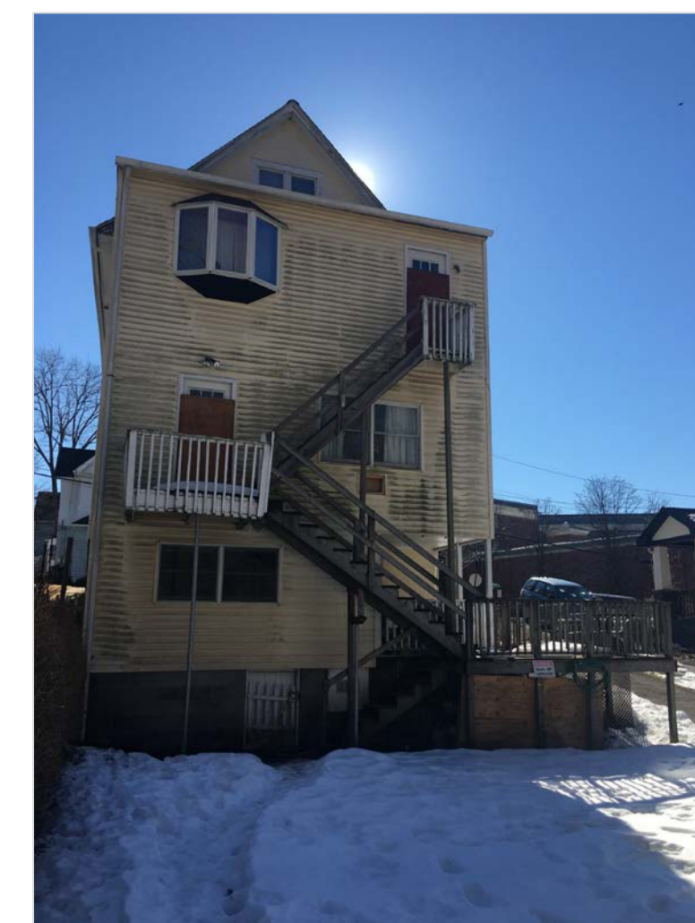
VIEW 3: EXTG FIRE ESCAPE/DECK
