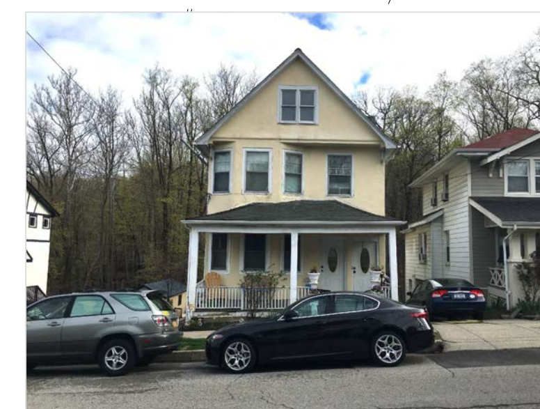
VIEW 6: FRONT FACADE
