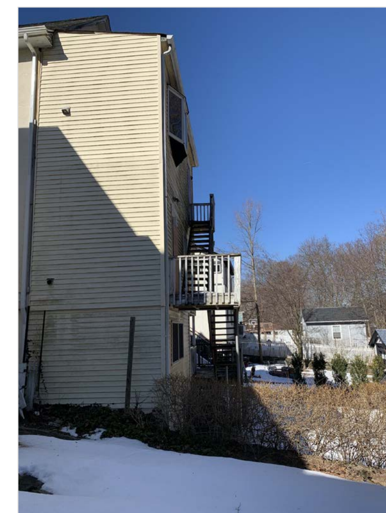
VIEW 4: FROM #67 HILLSIDE AVE REAR YARD
