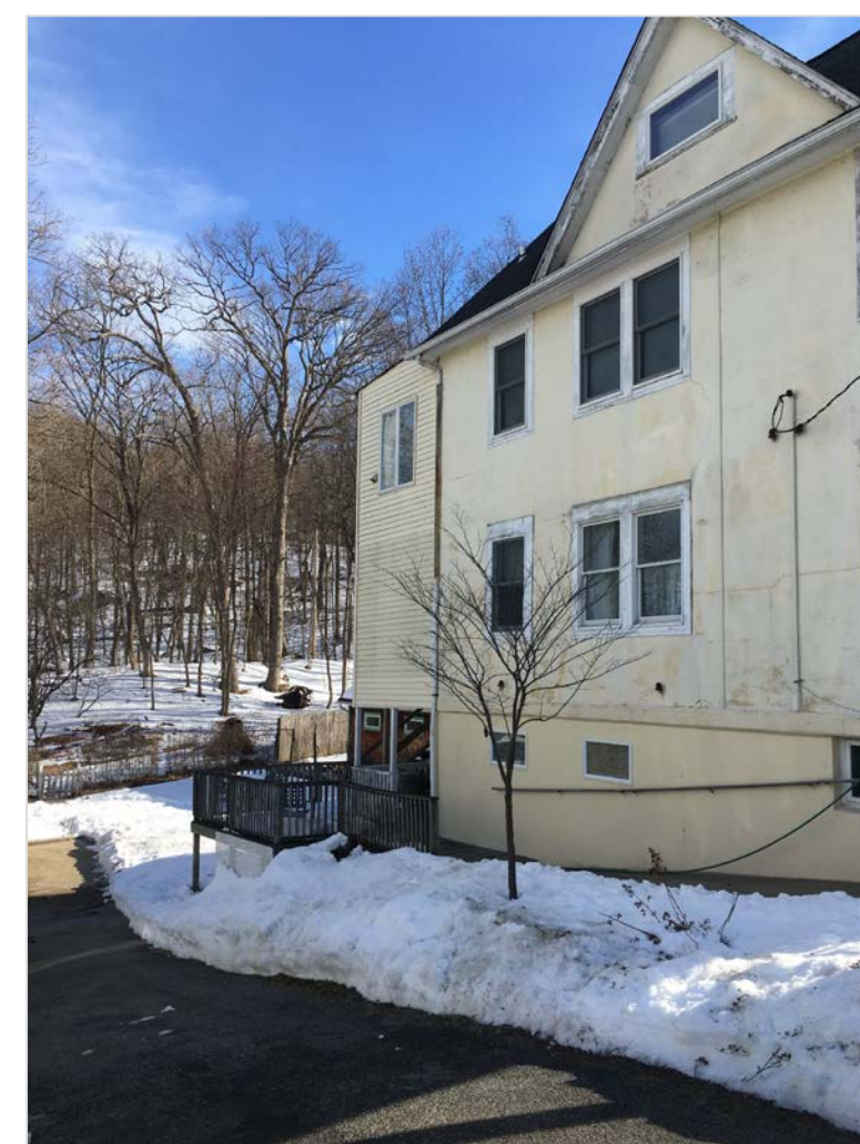
VIEW 2: WEST FACADE FROM HILLSIDE AVE
