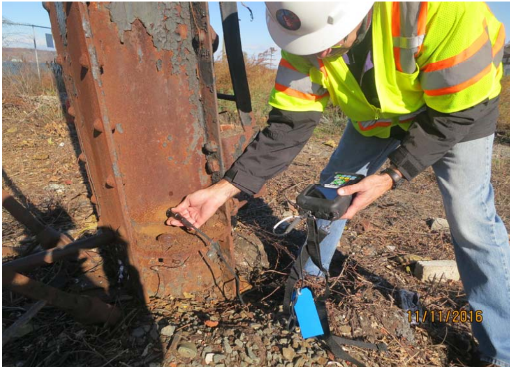
Photo No. 7: Northeast post exhibiting moderate corrosion. The layer of corrosion was removed from a testing location to record the thickness of the channel web, revealing approximately 10 percent loss of web area.
