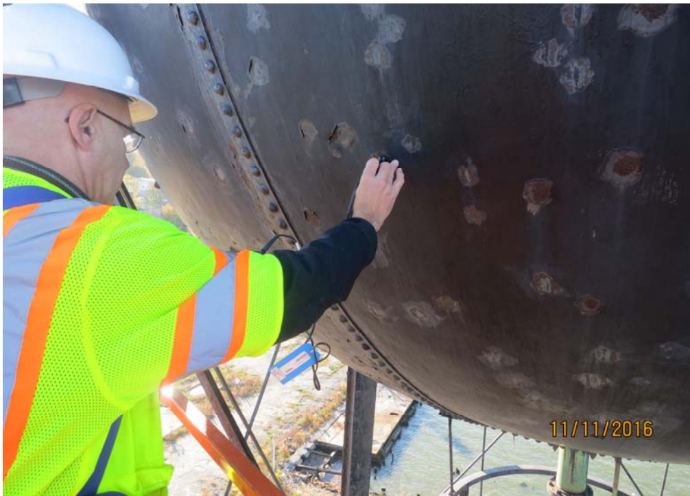
Photo No. 10: View of tank lower section exhibiting minor corrosion. Note recording of tank plate thickness using the ultrasonic measuring device.
