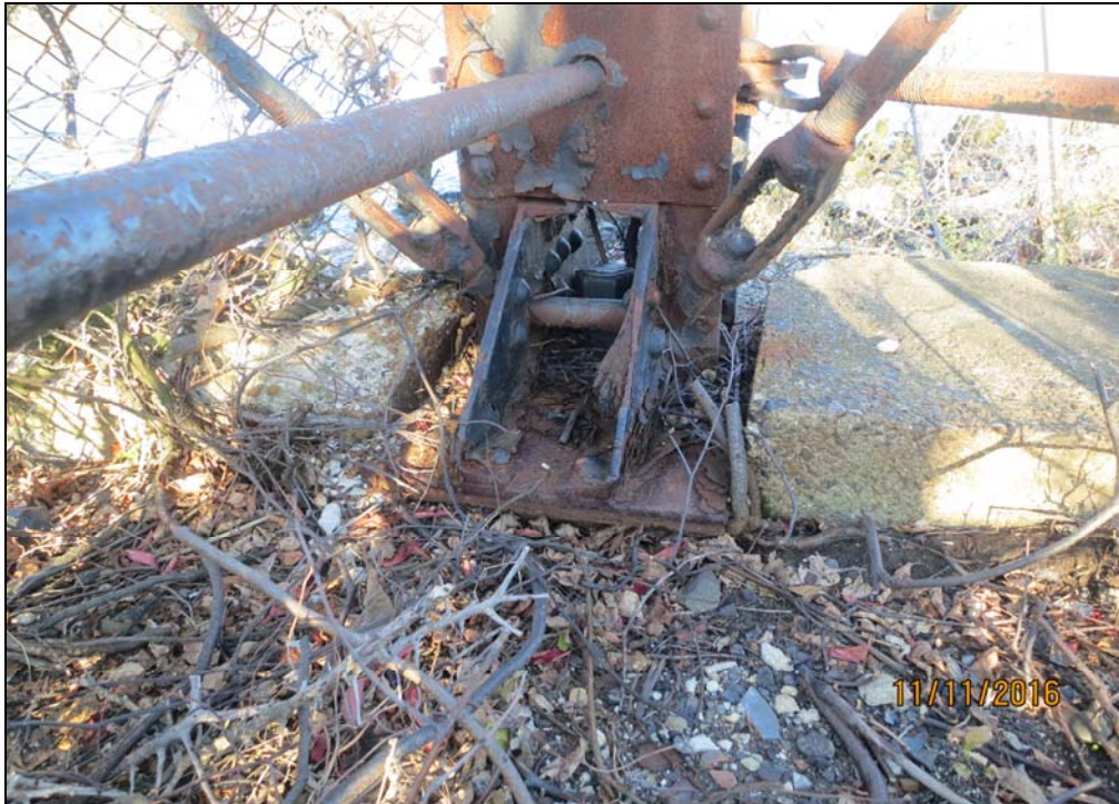
Photo No. 3: Northwest post anchor exhibiting moderate pack rust at the stiffener plates and moderate corrosion on the base plate. Note concrete foundation.
