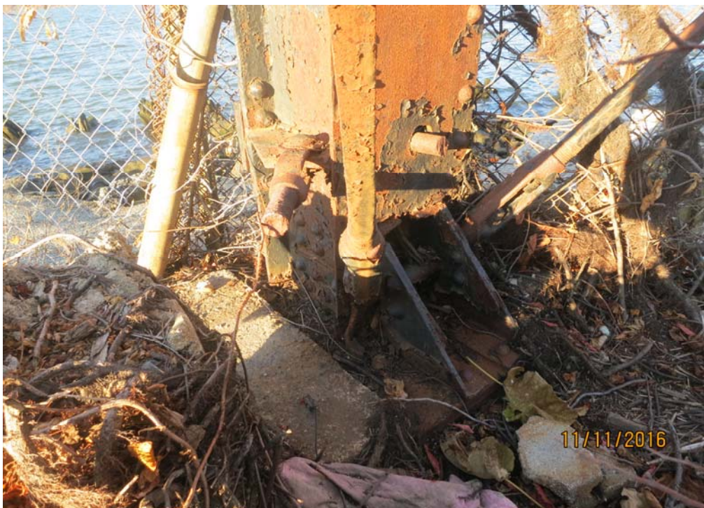
Photo No. 4: Southwest post anchor exhibiting moderate pack rust at the stiffener plates and moderate corrosion on the base plate.
