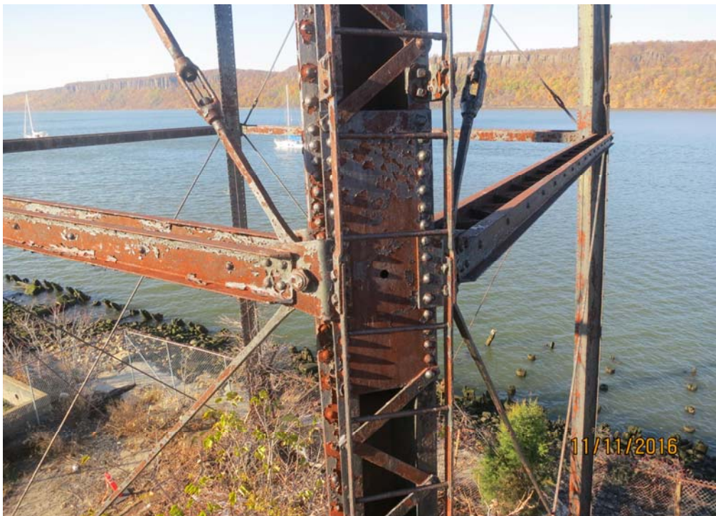
Photo No. 8: Typical post splice connection plates, struts bracing channels and cross rods exhibiting minor corrosion.
