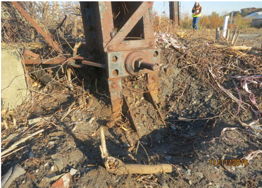
Photo No. 6: Southeast post anchor partially buried and exhibiting moderate corrosion on the stiffener plates.
