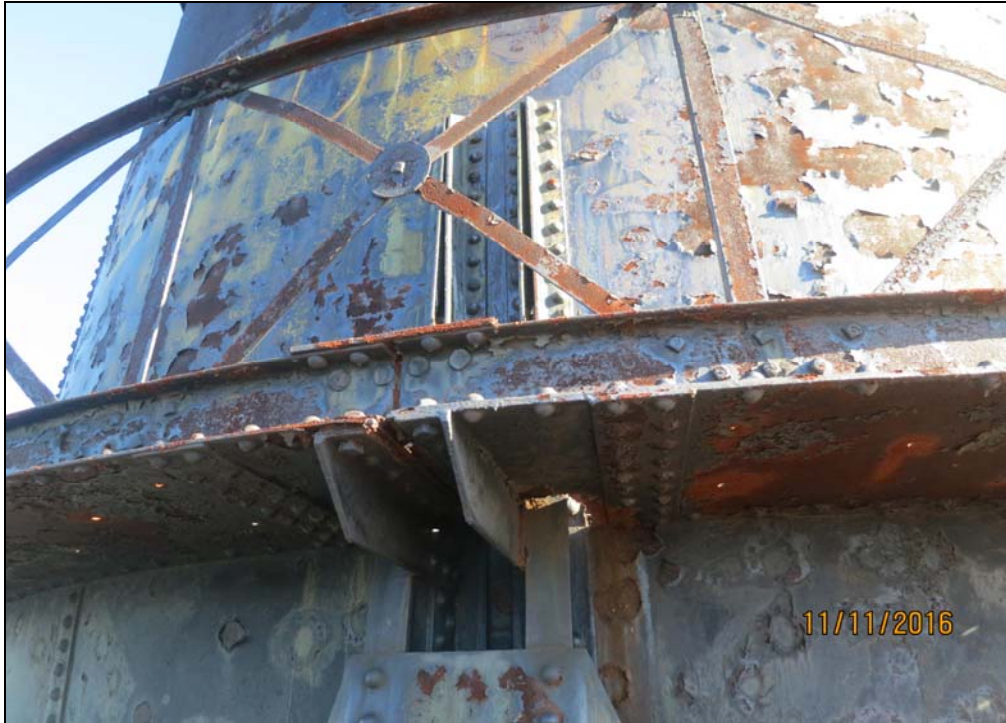
Photo No. 9: View of connection between tank and post in good condition.
