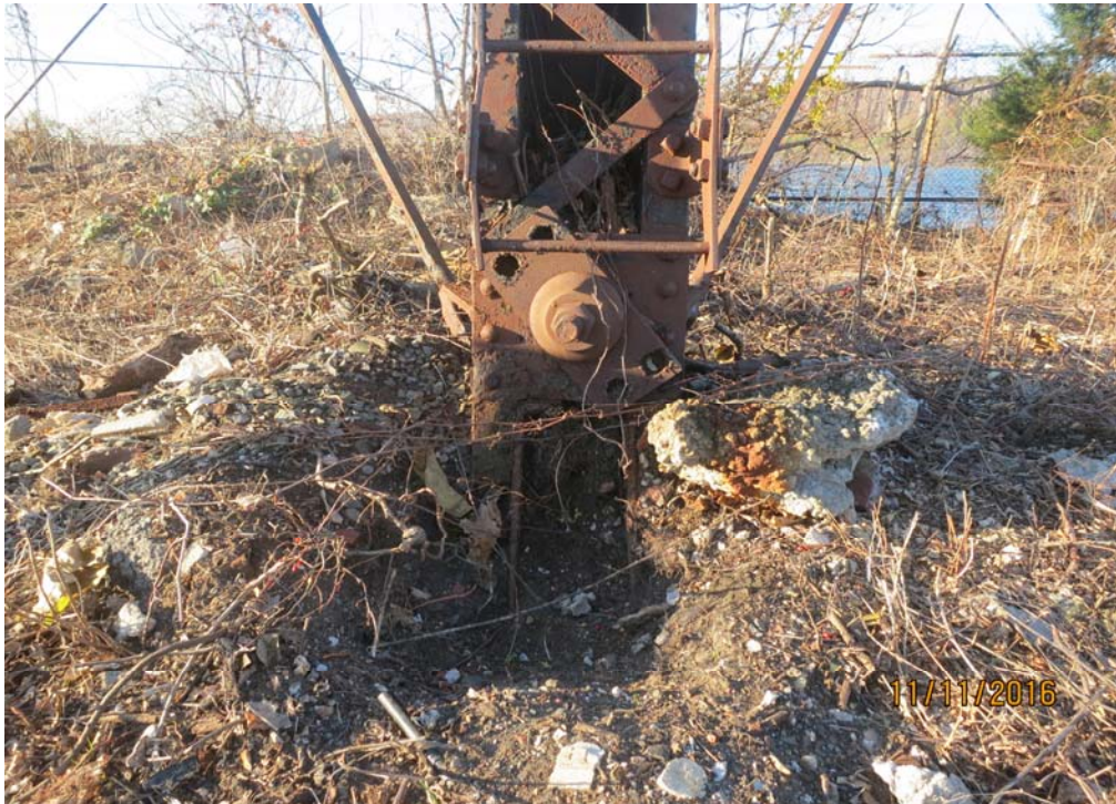
Photo No. 5: Northeast post anchor partially buried and exhibiting moderate corrosion on the stiffener plates.
