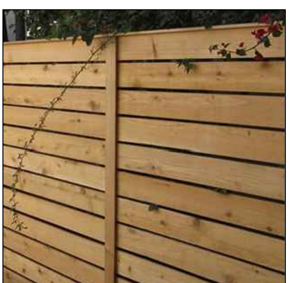
CEDAR FENCE HORIZONTAL STYLE, 6 FT HGT. 1"X6" BOARDS, 4X4 POSTS TO MATCH NEIGHBOR'S FENCE
