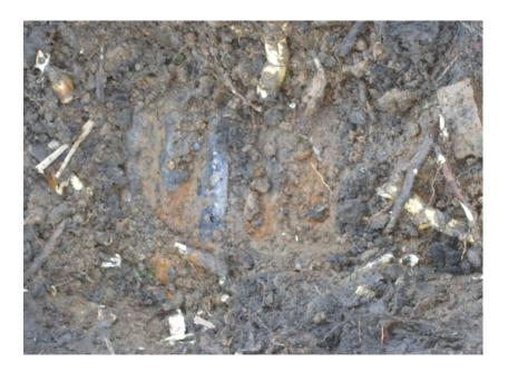
Photo 2: Exposed portion of 42" piping at berm around 2.5' below ground surface
