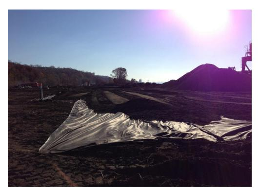
Photo 4: Looking south, observing filter fabric and fill material
