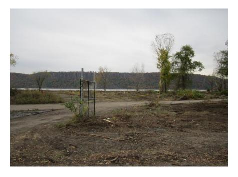
Photo 2: Site grubbed. Few large trees left to be removed with excavator
