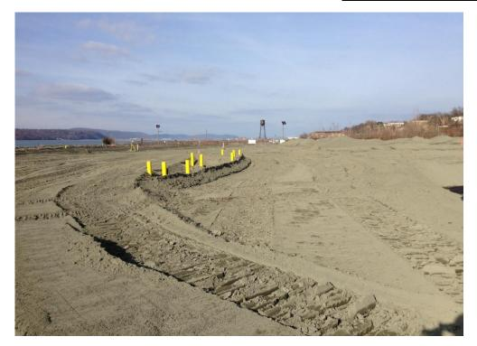
Photo 3: Looking north, observing placement of clean fill material
