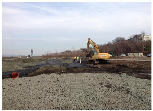
Photo 4: Looking north, observing the laying of new fabric
