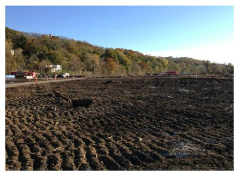
Photo 3: Looking southeast, showing recently graded and grubbed surface
