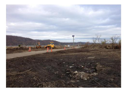
Photo 2: Looking northwest, the bulldozer begins rough grading the site
