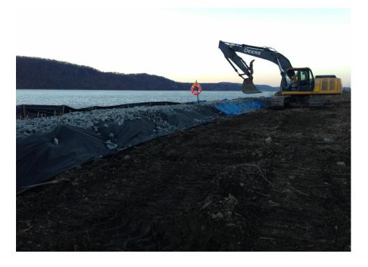
Photo 4: Looking NW, temporarily stabilized berm
