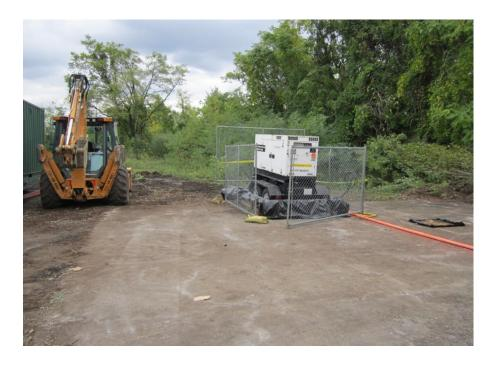
Photo 2: Generator and containment around unit
