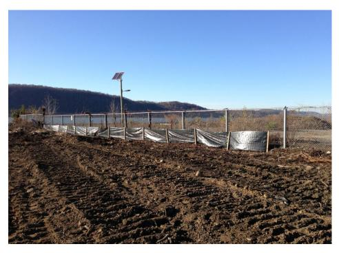
Photo 4: At the northern border of site, showing silt fence installed to protect the swale, prior to nor'easter
