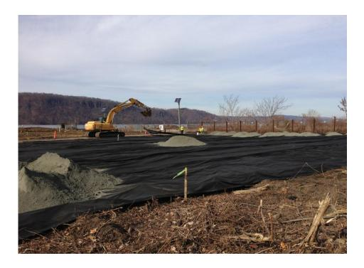
Photo 2: Looking northwest, observing the placement of filter fabric
