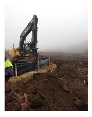
Photo 2: Looking north, observe construction of silt fence and hay bales along river's edge
