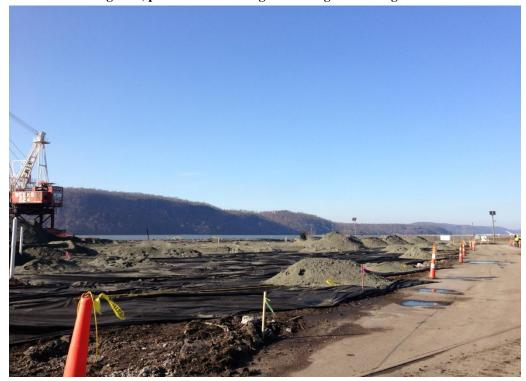
Photo 2: Looking west, observe grading and spread of new material over filter fabric
