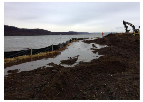
Photo 1: Looking NNW, observing breach of sediment control measures, due to extreme high tide
