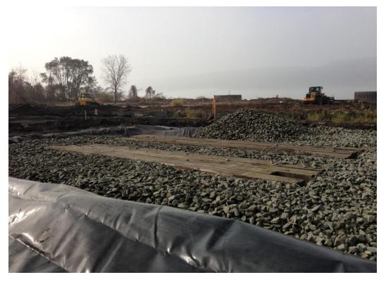
Photo 4: Looking SW, showing the construction of the de-con pad
