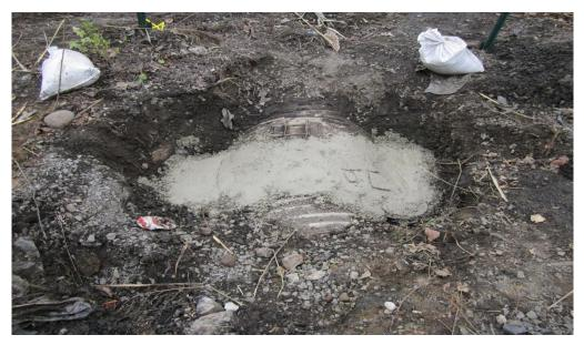
Photo 2: Collar and breach cemented
