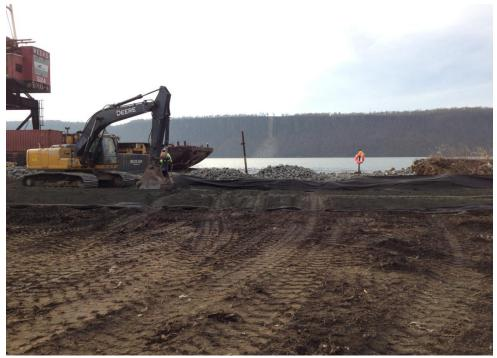
Photo 3: Looking west, observing the newly spread out material atop filter fabric, with berm repair
