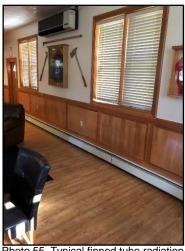
Photo 55. Typical finned tube radiation
