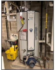
Photo 44. PVI DHW heater and storage tank
