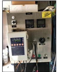
Photo 81. Typical pool chemical monitoring system
