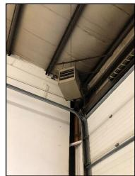
Photo 93. Typical gas-fired unit heater abandoned in place
