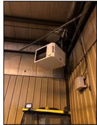
Photo 90. Typical gas-fired unit heater serving garage
