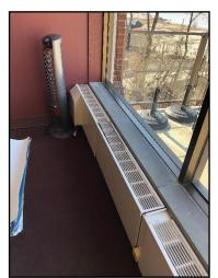
Photo 11. Typical finned tube radiation
