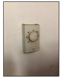
Photo 92. Thermostat controlling electric baseboard
