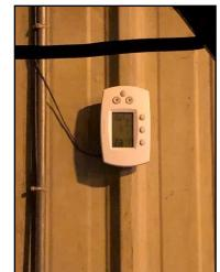
Photo 94. Thermostat controlling gas-fired furnace Photo
