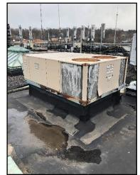
Photo 14. Packaged Trane RTU serving courtroom
