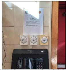
Photo 77. Timers appear to be for exterior lighting
