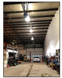
Photo 98. Typical metal halide light fixtures
