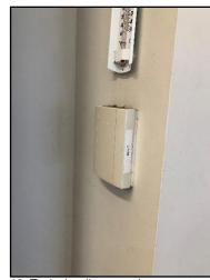
Photo 12. Typical wall mounted temperature sensor
