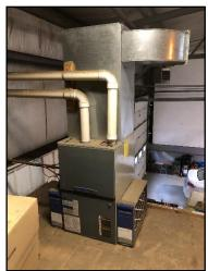
Photo 89. Gas-fired furnace serving repair shop
