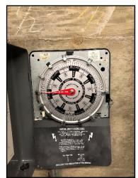
Photo 30. Typical timer for exterior lighting
