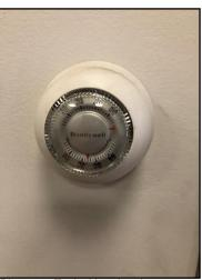
Photo 56. Typical heating thermostat
