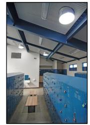
Figure 49. "Solatube" skylight installed in locker room
