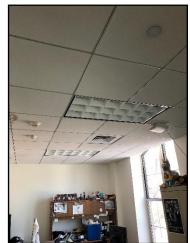
Photo 45. Typical 32W T8 lighting fixtures in offices
